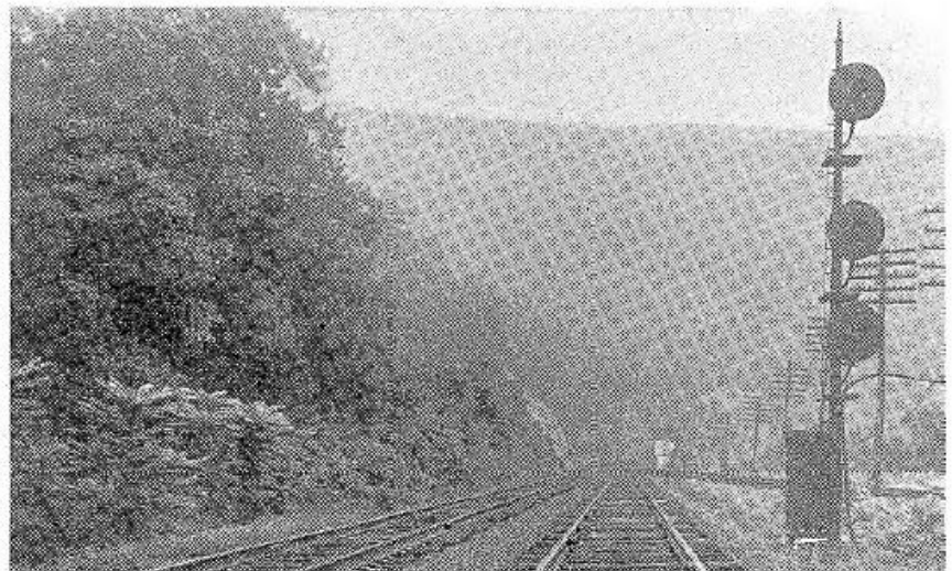
Above—Plug in type polar switch repeater relays Below—Typical searchlight type home signals
