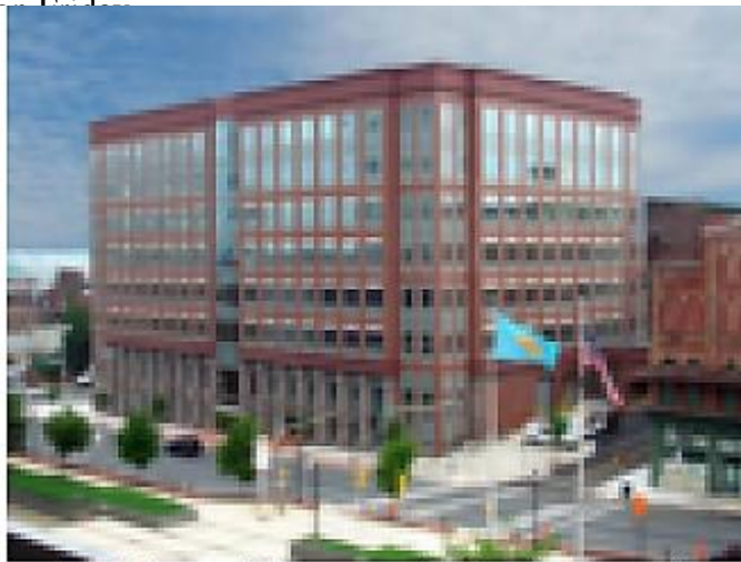
Amtrak has named the contractor for the project to create its Unified Operations Center in Wilmington, Del. (Photo by Tevebaugh Architecture)
